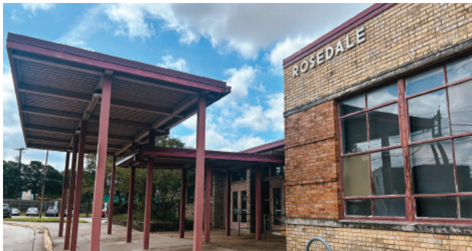
The former Rosedale Elementary building
