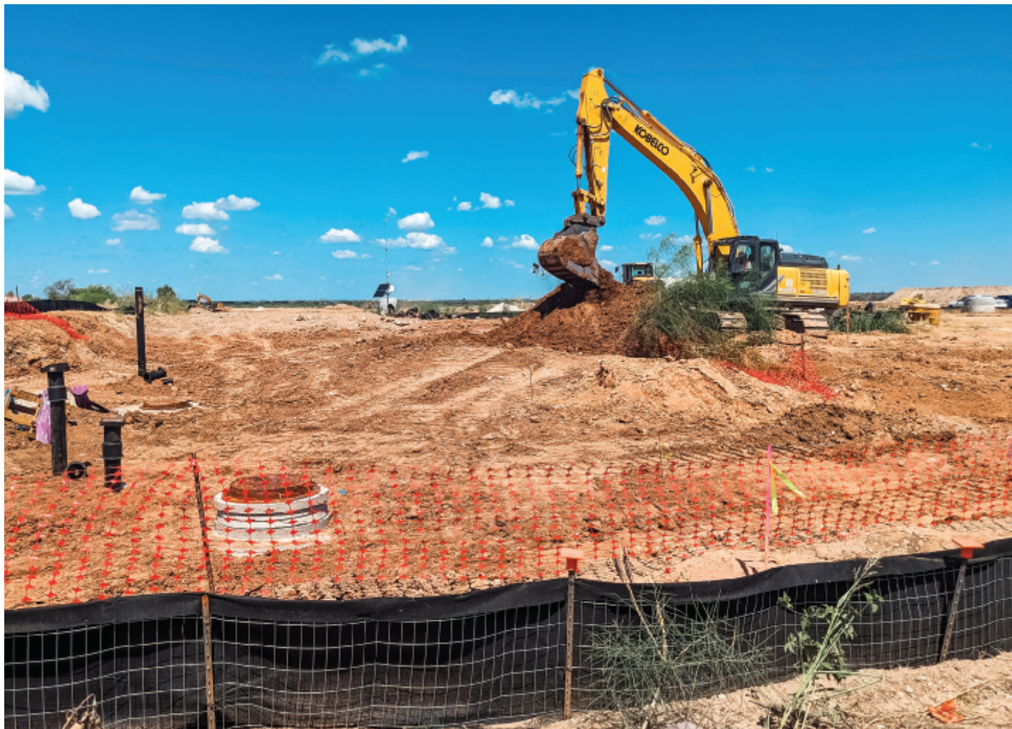
Construction activity at Dog's Head area
