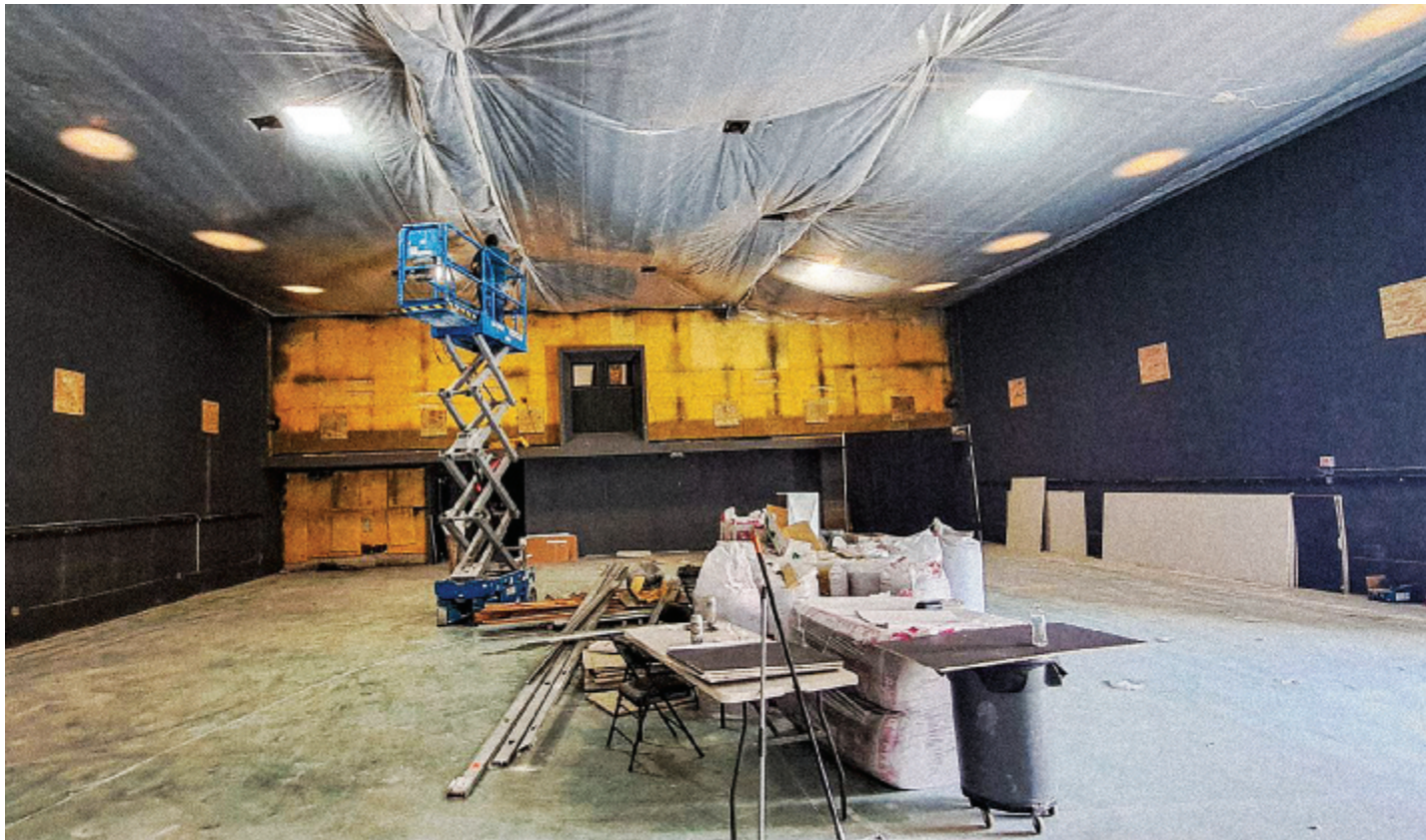
The under-construction site of AFS Cinema's third screen, slated to open later this year
