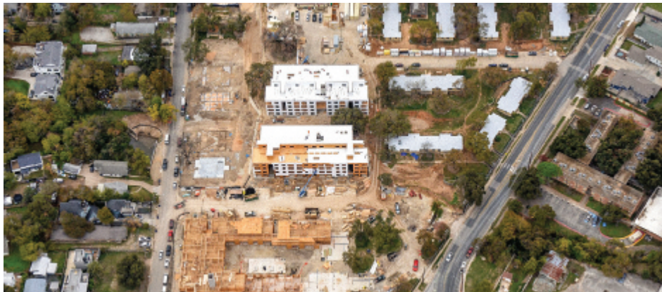
Rosewood Courts construction
