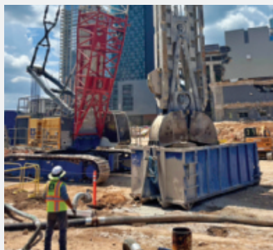
Austin Convention Center construction
