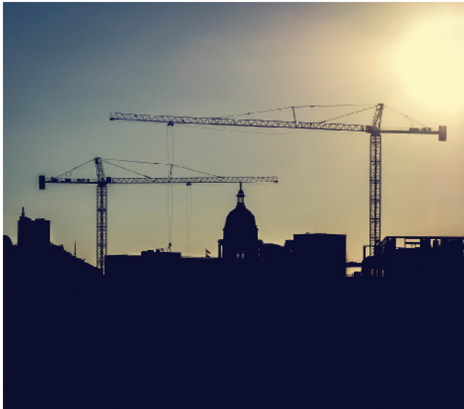
Construction in Austin in the heat
