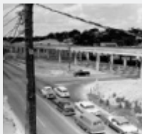
I-35 construction at Sixth St. in 1960 VIA TEXASFREEWAY.COM
