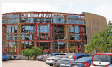
Demolished Frank Erwin Center PHOTO BY LARRY D. MOORE / CC BY 4.0
