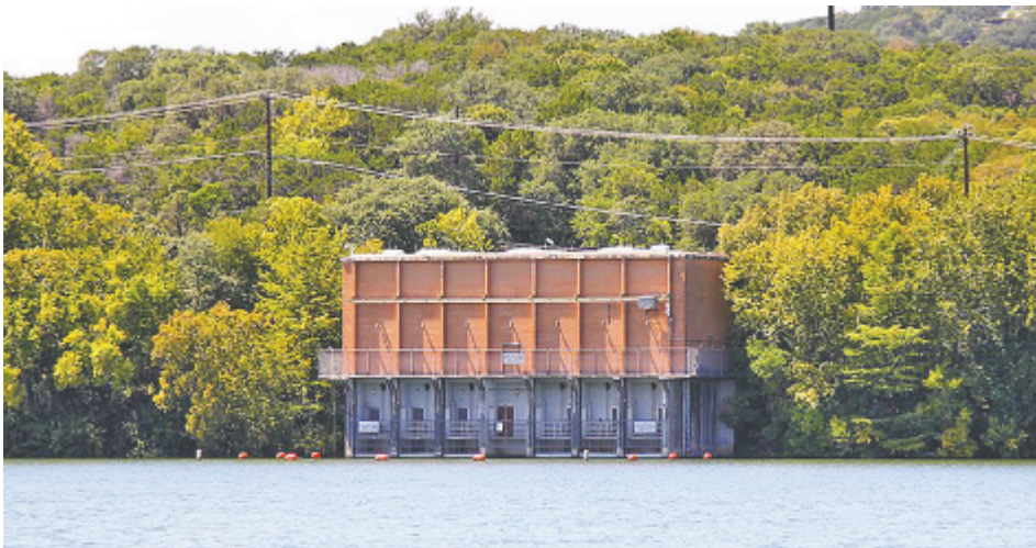
The troubled Ullrich Water Treatment Plant on Lake Austin
