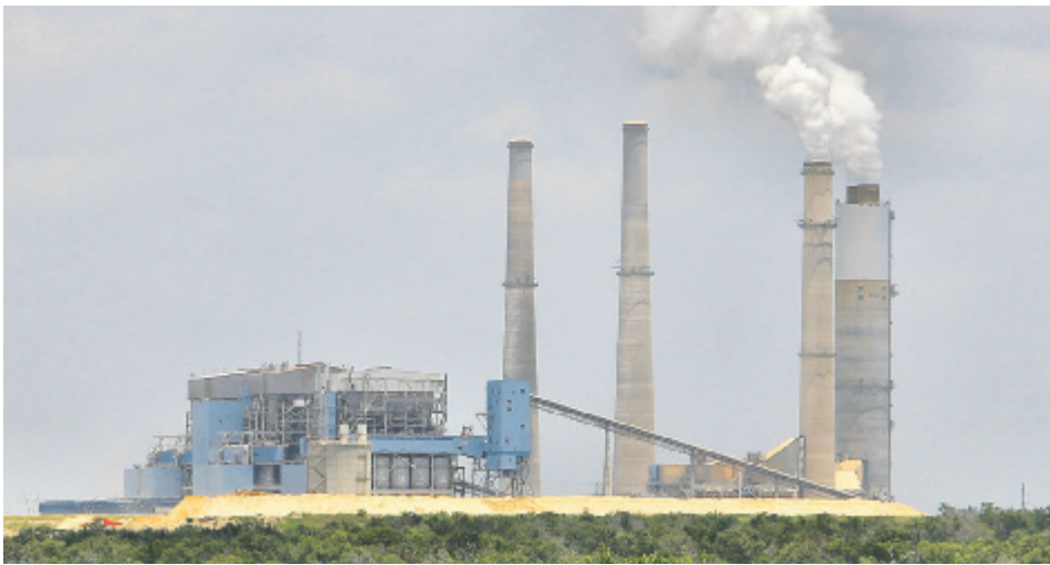
The Fayette Power Project near La Grange produces 72% of Austin Energy's carbon emissions, but only generates 13% of AE's total power
