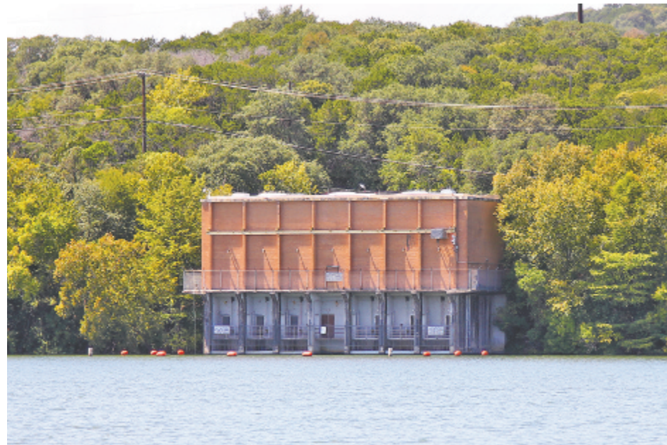
The troubled Ullrich Water Treatment Plant on Lake Austin
