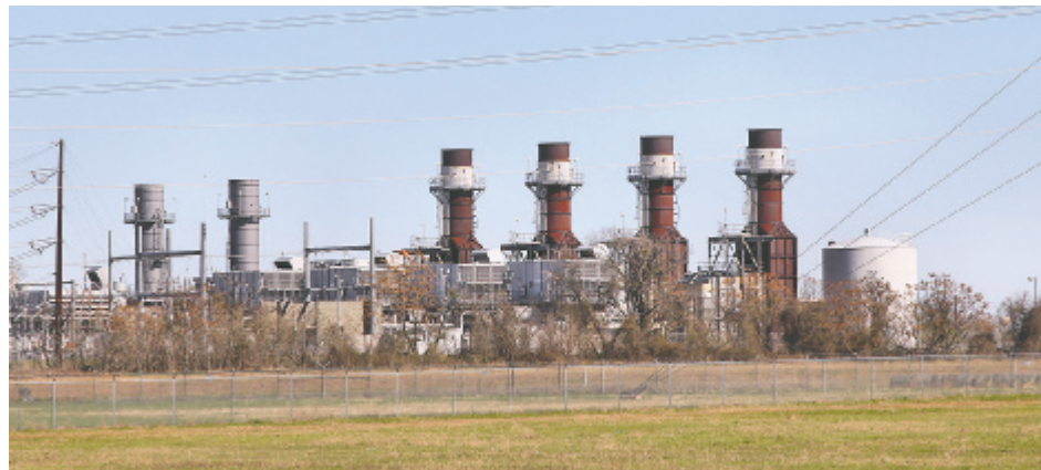
Austin Energy's Sand Hill Energy Center power plant
