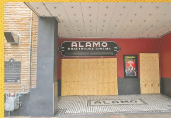
The Alamo Ritz, boarded up in 2020 JOHN ANDERSON
