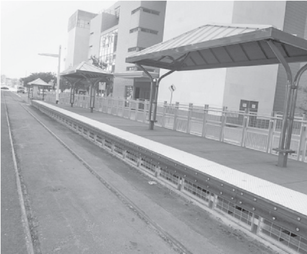
Capital Metro recently completed its Downtown MetroRail station, located a stone's throw from the Convention Center, in preparation for the transit agency's Red Line services set to roll out early next year.
