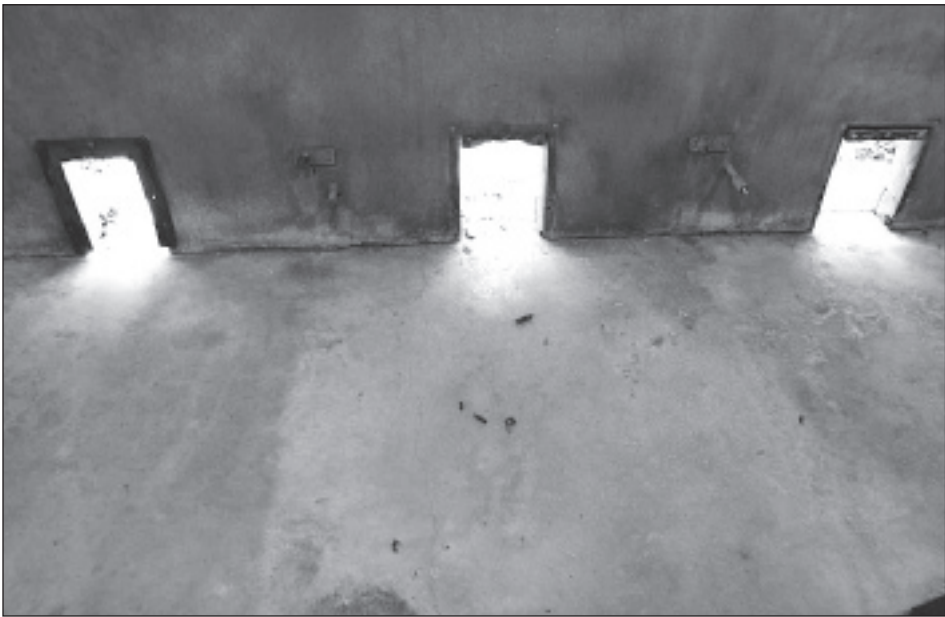
After Theisen-Watt relocated a group of dogs to Houston, PPI’s staff and volunteers demolished the cramped and dark kennel. The area will now be used as a kitchen and laundry room.
