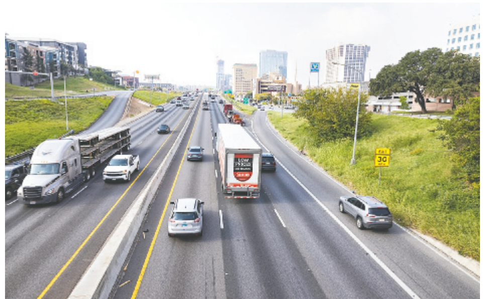
I-35, looking south from the 12th Street overpass
