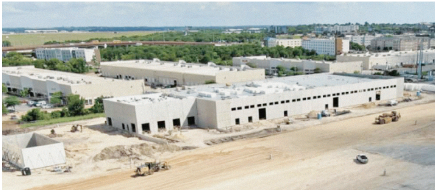
The Marshalling Yard and warehouse in 2021
