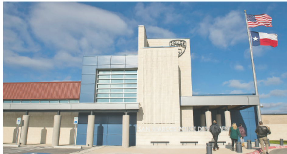
San Marcos Police Headquarters
