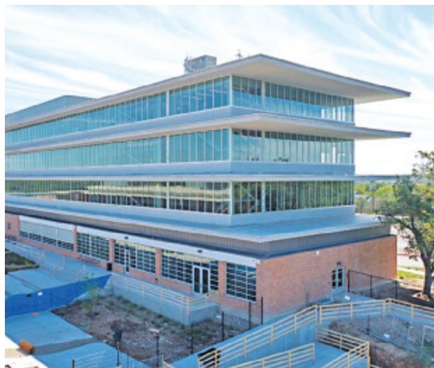
Construction at Eastside Early College High School, funded by the 2017 bond
