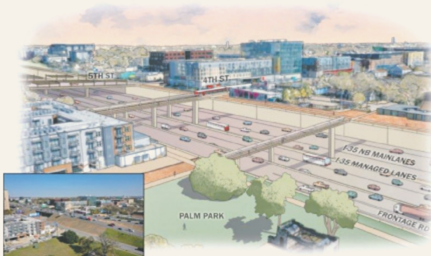
A rendering of “Improved” I-35 bridge crossings at Third Street Downtown, showing the depths of the highway below. This is a stretch where deck plaza “enhancements” would cover the mainlanes, should they be constructed, converting this ditch into an effective linear park.
