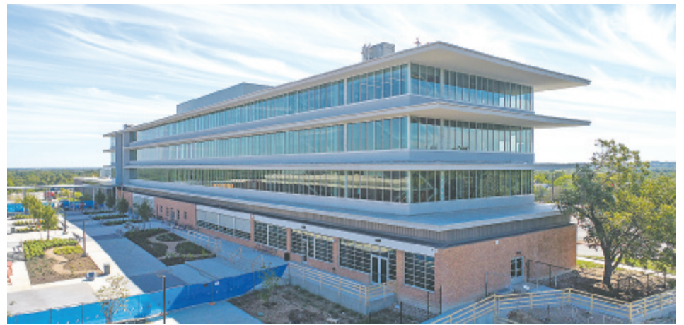
Construction at Eastside Early College High School, funded by the 2017 bond
