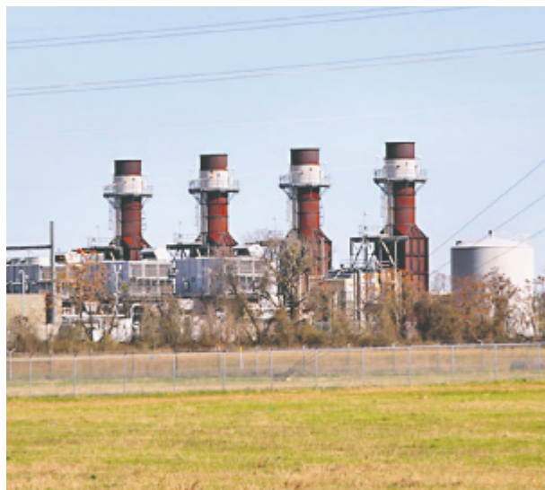
Austin Energy's Sand Hill Energy Center power plant
