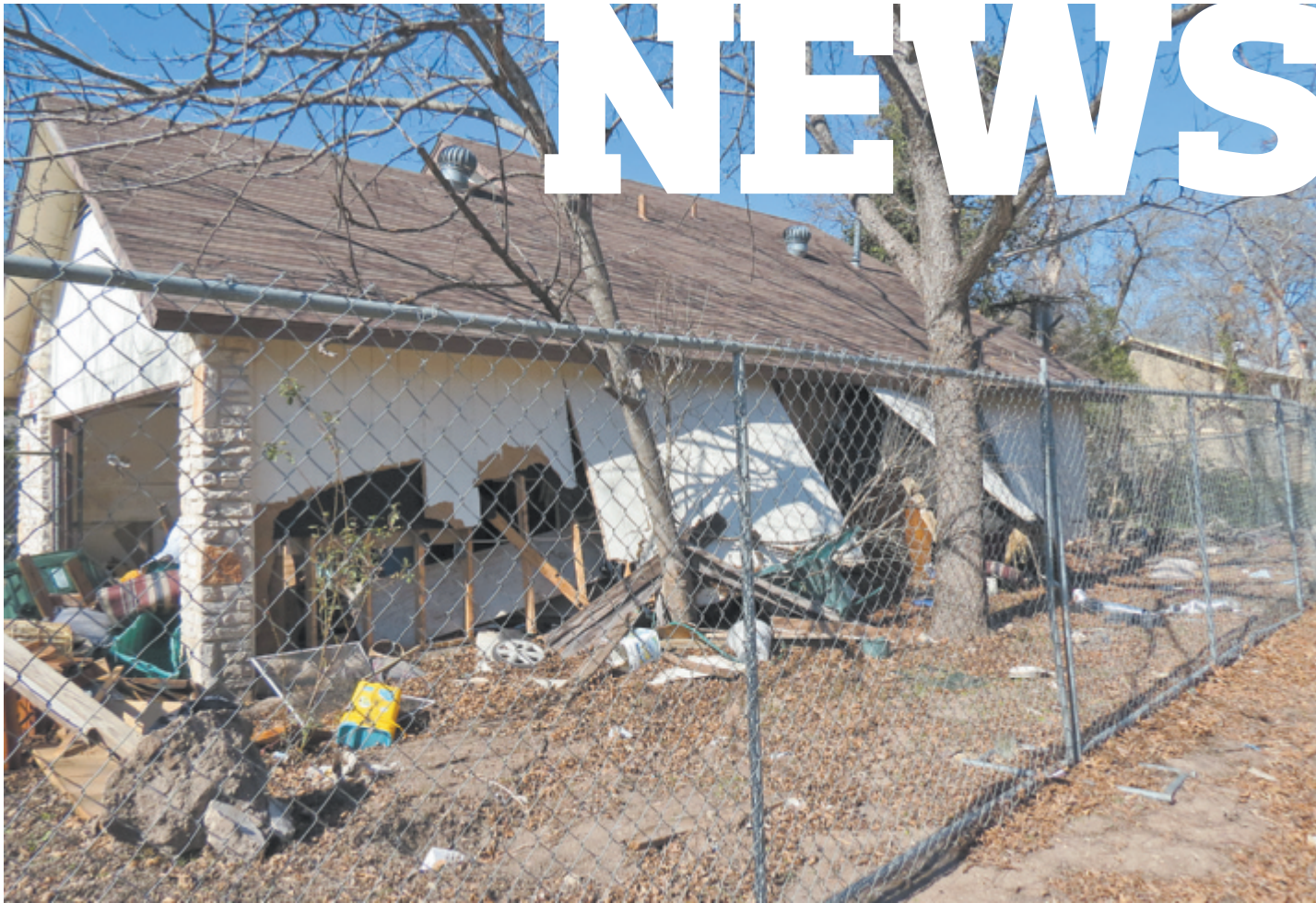
A familiar sight in the Onion Creek neighborhood – a home destroyed by the flood, surrounded by a chain link fence, and waiting to be demolished.
